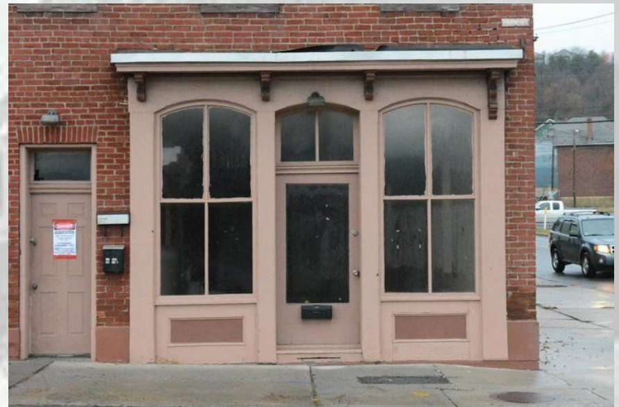
Good example of “Bulkhead” -recessed wood panels with wood trim.
