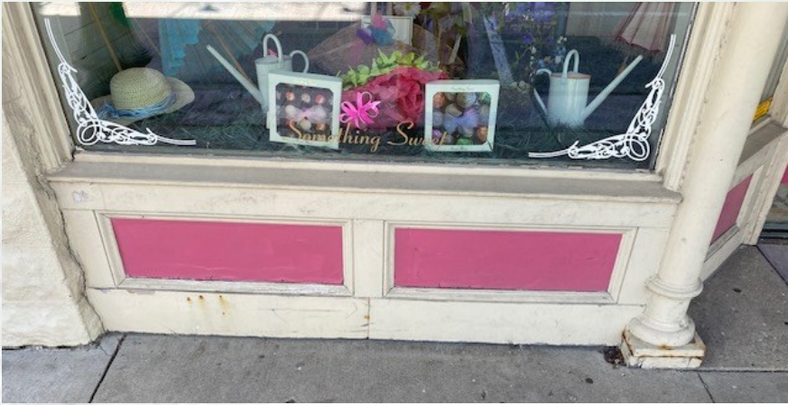
Good example of bulkhead— existing store on Main Street
